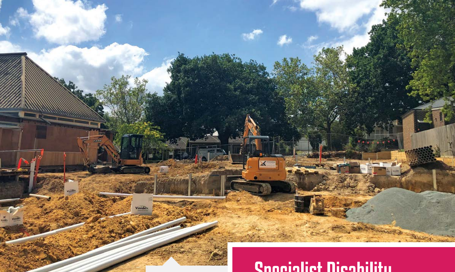
Photo: Progress at our Anderson Street site.
